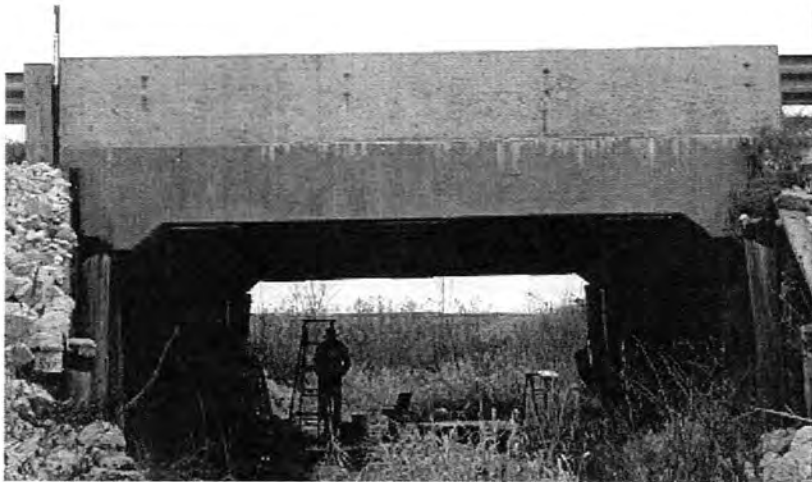
b. Side view of bridge.
