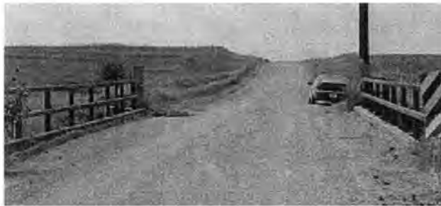
c. End view of bridge.
