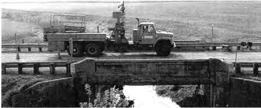
b. Side view of bridge.
