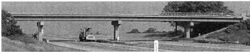
c. Side view of bridge.
