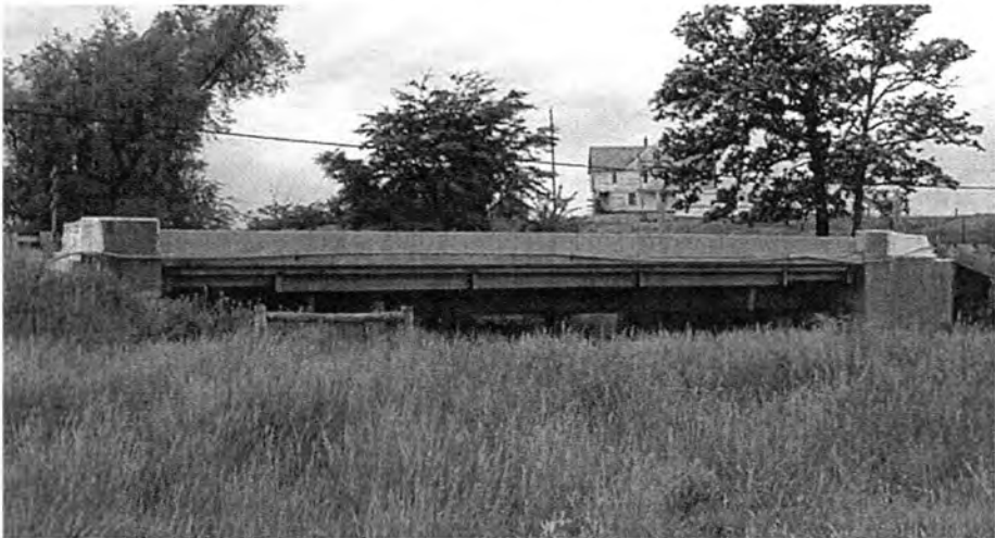
d. Side view of bridge.
