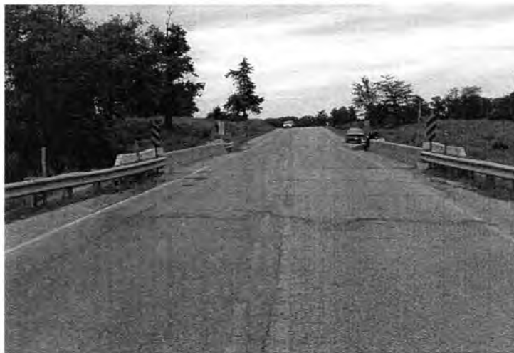
a. End view of bridge
