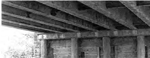
b. Girders and the West side of abutment.
