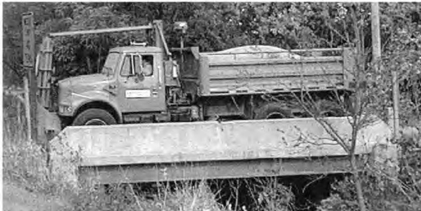
b. Side view of bridge
