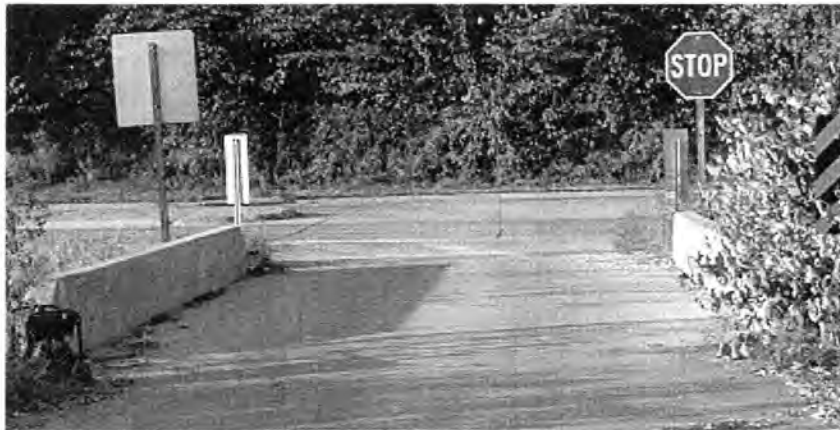
a. End view of bridge.
