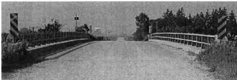
d. End view of bridge.
