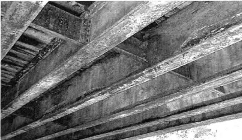
b. Girders on East side at midspan.
