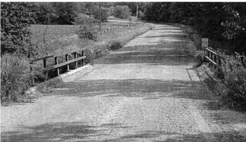
c. End view of the bridge.
