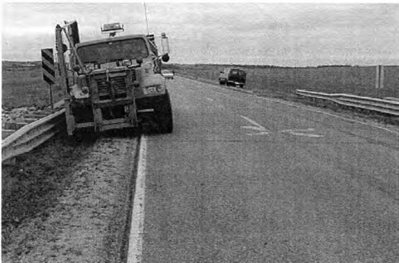
c. End view of bridge with truck path Y4.
